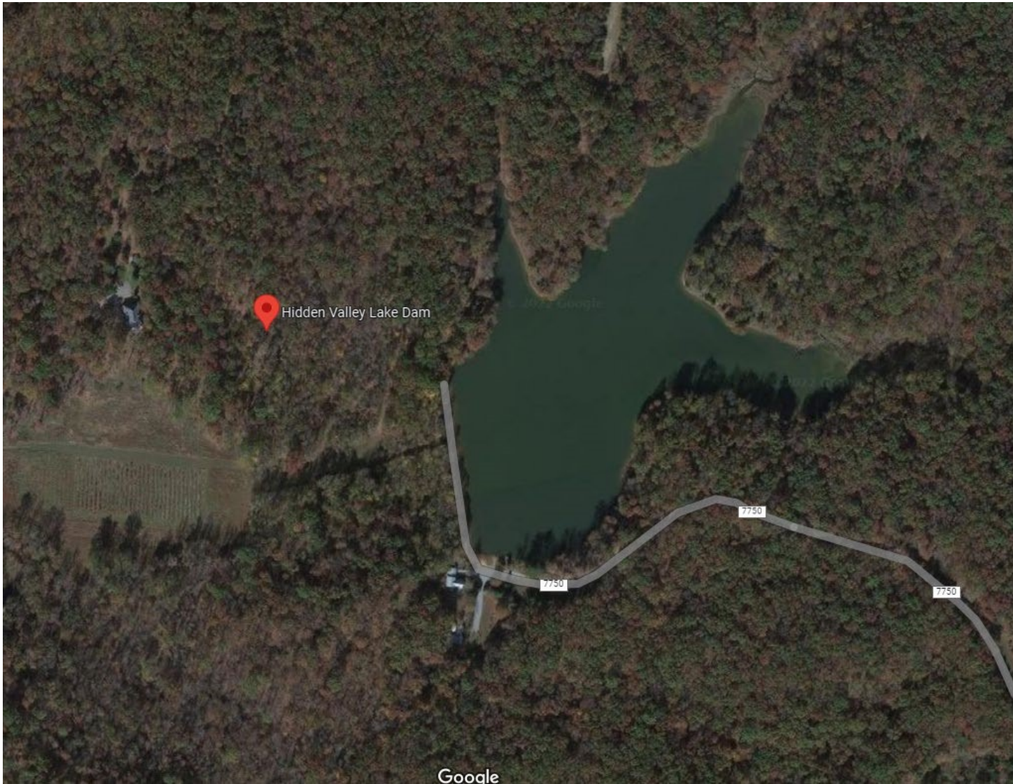
Hidden Valley Lake Dam: is considered a is a Class “A” Low Hazard the Dam located 3.7 miles from Wynne.
