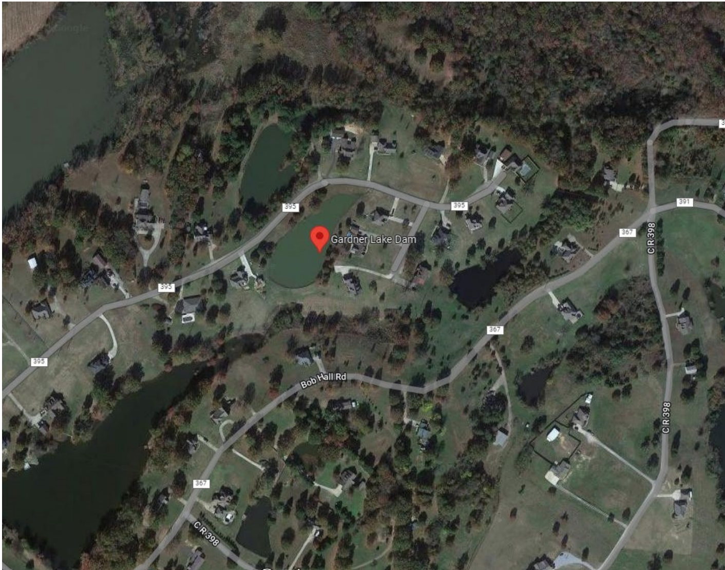
Gardner Lake Dam: is considered a Class "B" Significant Hazard dam considering the number of residents surrounding the Dam.
